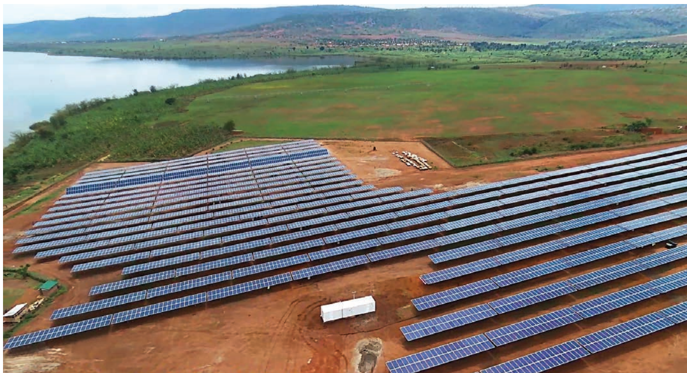
This 3.3 MW solar plant in Rwanda's Bugesera region powers 63 center pivots and required pump stations, benefitting more than 2,000 farm families from the NASHO cooperative. Ultimately, the excess power from this solar plant will be sold back to the grid.
